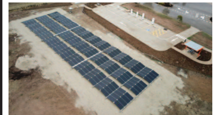
AN ELECTRIC VEHICLE CHARGING STATION IN ALBURY-WODONGA MADE BY THE MODULAR PANEL MANUFACTURING COMPANY 5B. THE COMPANY SAYS ON ITS WEBSITE THAT THE INSTALLATION TOOK A MORNING'S WORK BY A TEAM OF TWO.
